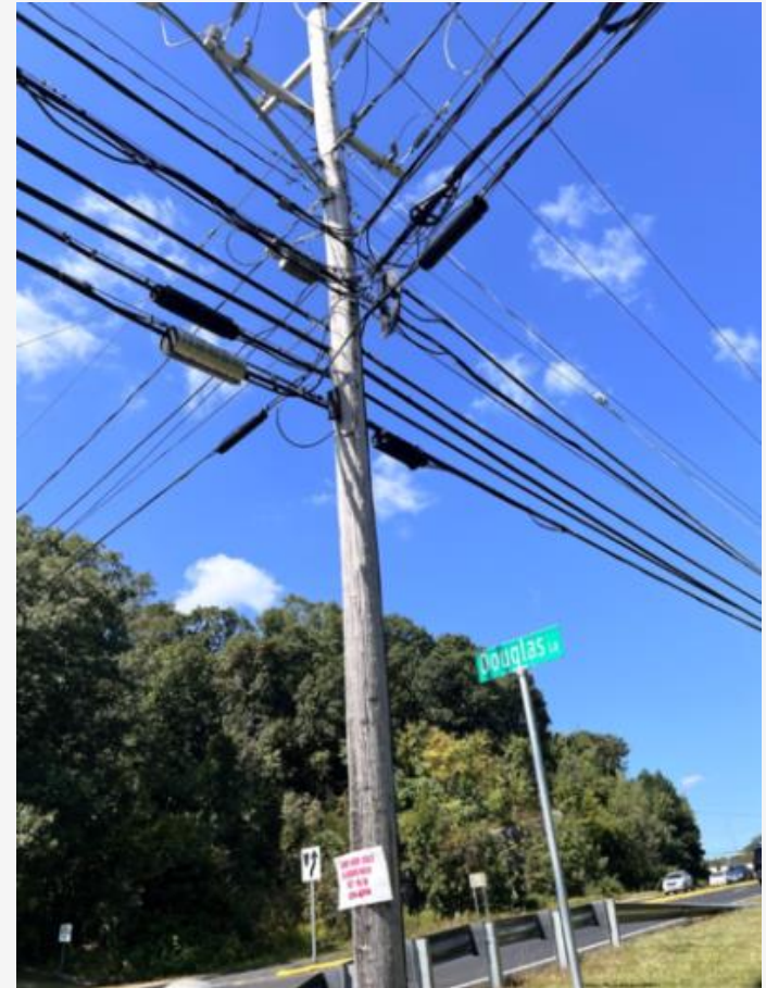
Typical Aerial Cable Installation and Splice Enclosure
