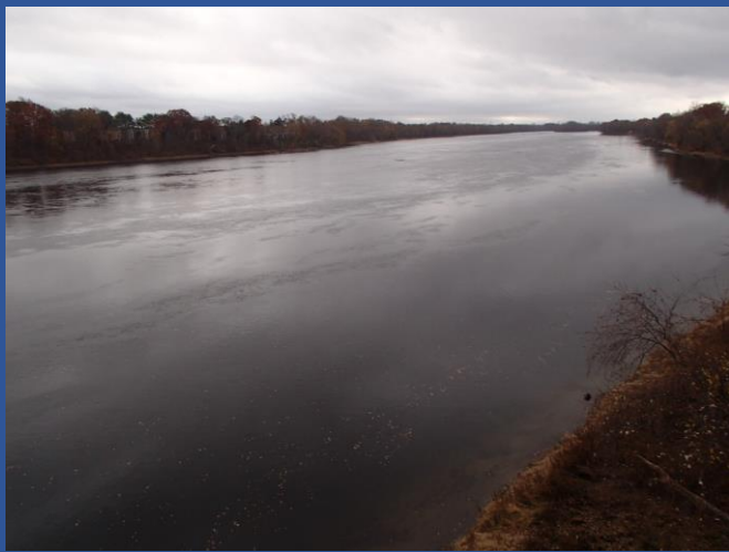
Channel downstream of bridge, looking South.
