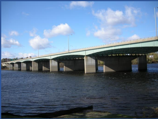
Channel under bridge, looking North.
