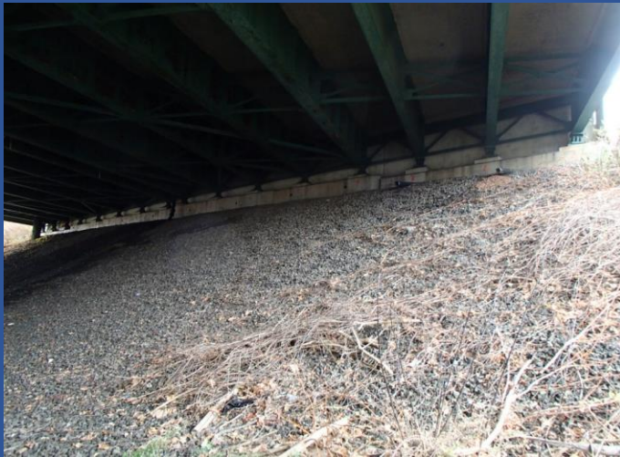
Abutment & slope protection typical condition (Abutment No. 1).
