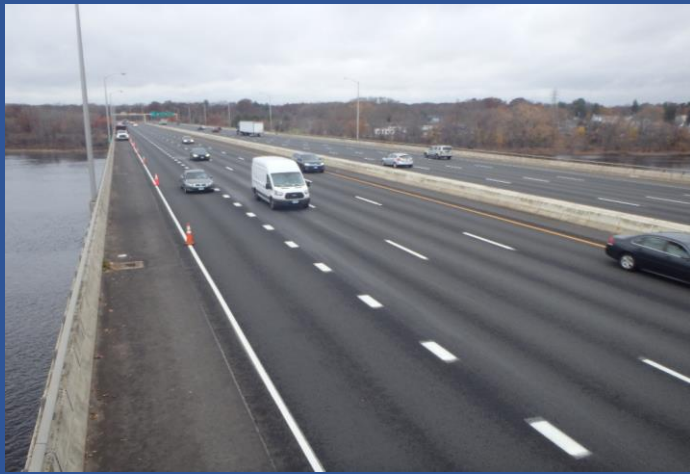
Top of Bridge looking West.
