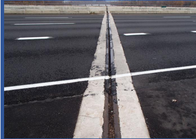
Strip seal expansion joint at Pier 7
