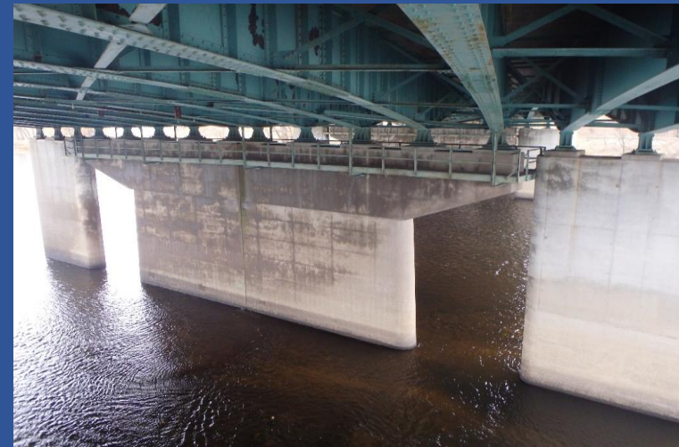
Pier typical condition (Pier 9). (Note: outside stems for widened bridge)
