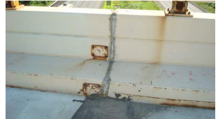
Safety Walk and Parapet
