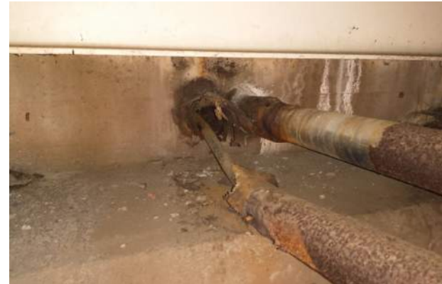
South Abutment – West Lines Rehabilitation of Bridge No. 01164 // State Project No. 0080-0312
