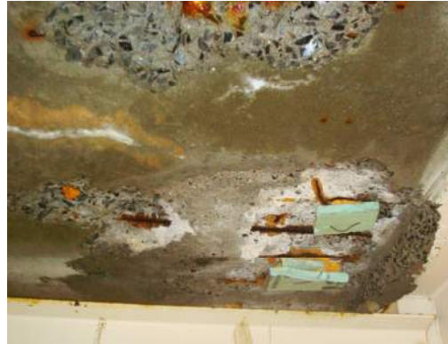
Underside of Deck
