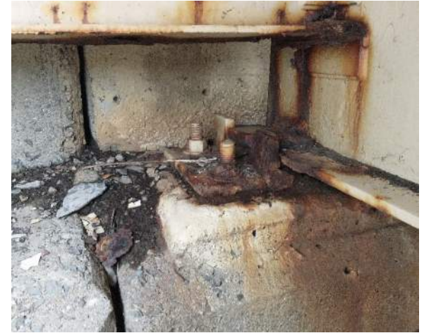
Bearing condition at Abutment
