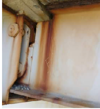
Pin & Hanger Assembly and Stringer End
