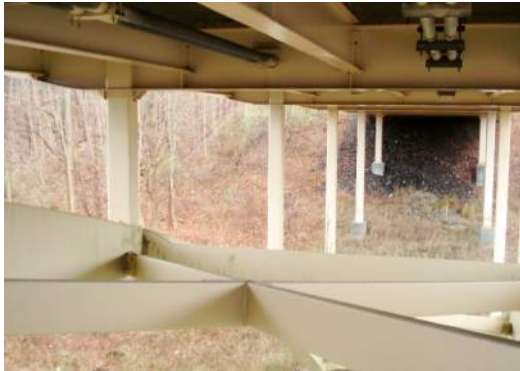
Arch Column, Floor beam, and Stringers
