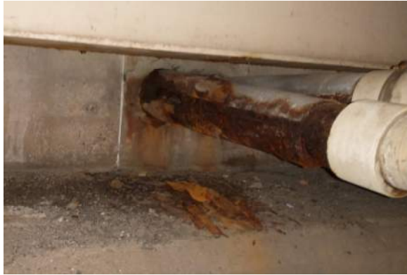
North Abutment – West Lines
