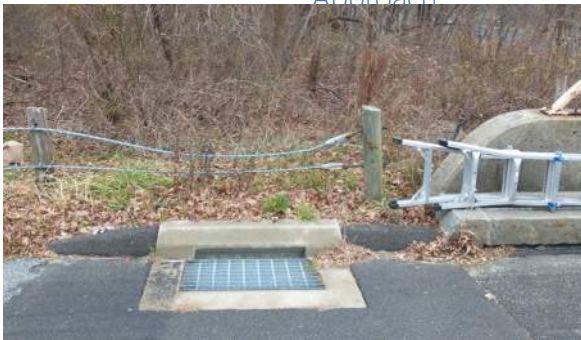
Transition – Approach Guiderail to Bridge Endblock
