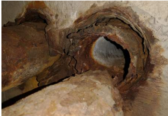
South Abutment – East Lines
