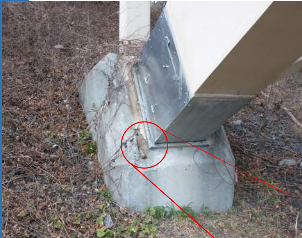
Arch Rib Abutment
