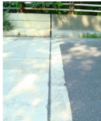
Strip Seal at Abutment
