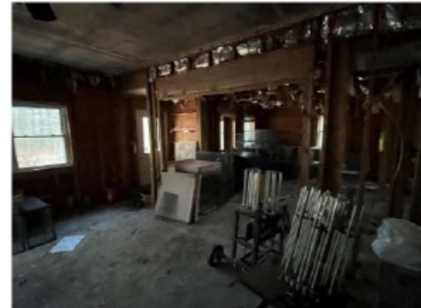
Existing Care- Taker's Lodge
