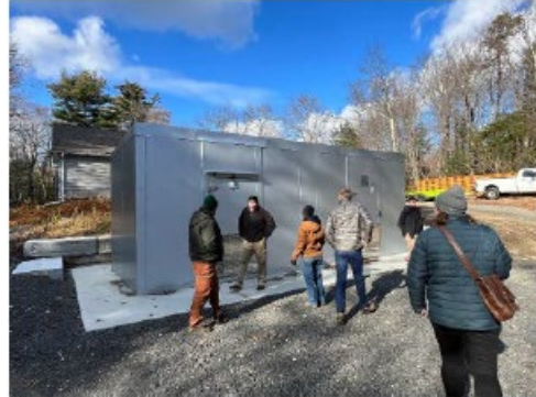
Existing Walk-in Freezer
