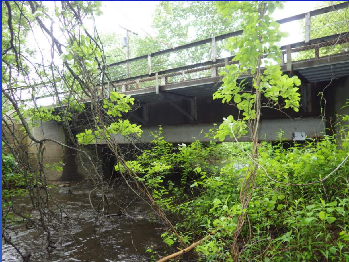
North Elevation (Looking Downstream)
