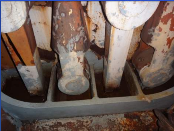
Counterweight Rope Connection
