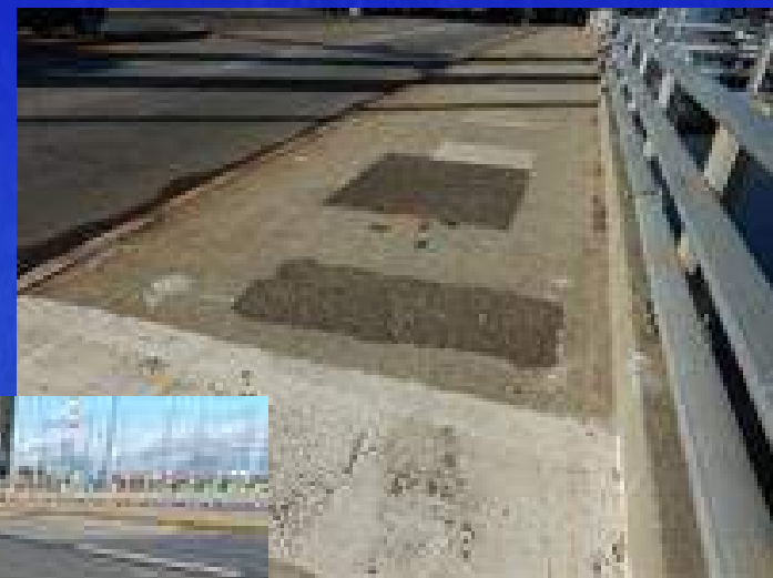
Patching along north sidewalk
