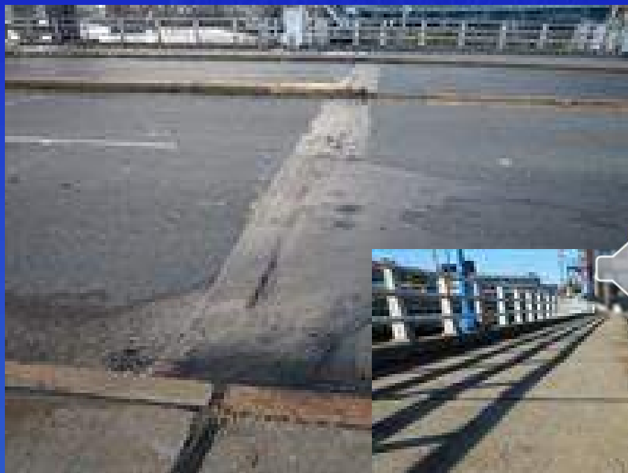
Pier 4 roadway joint
