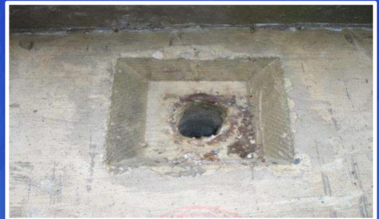
Missing Post tension Anchorage and Transverse Tie
