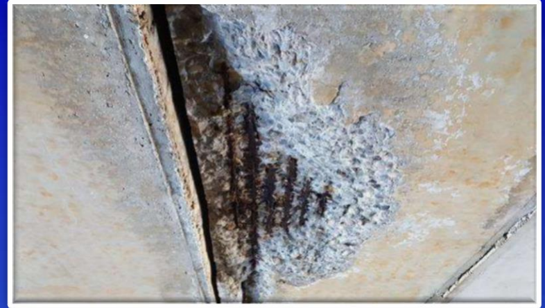
Large Spall with Severed Strand
